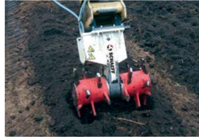
SOIL PREPARATION / MIXING
